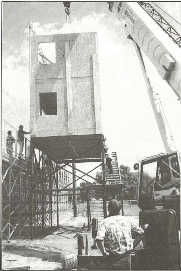
Raising the press box was one highlight of the project. Photo by DennisNoe.
