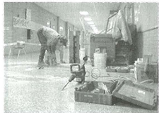
The early stages of the emblem installation. Photo by Andrew Fotenakes
