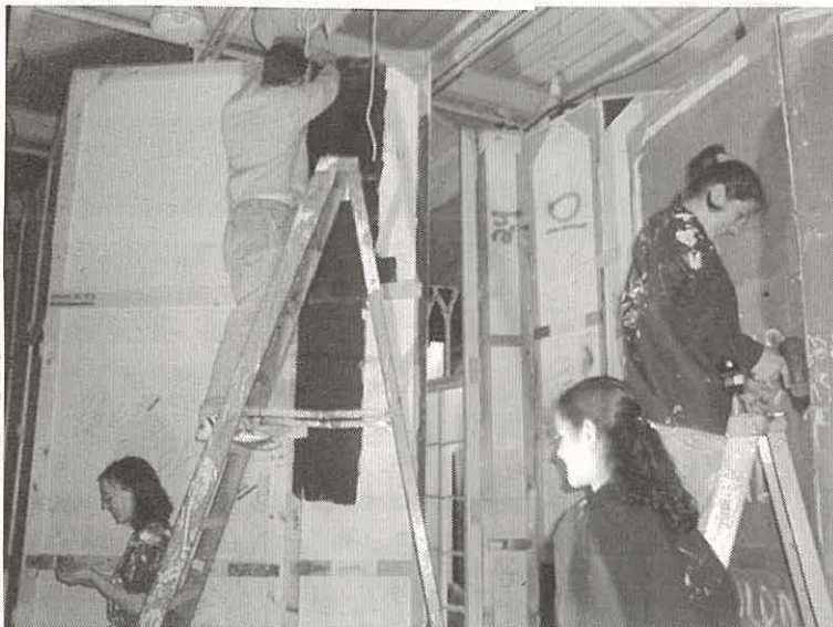
⊙ Jamie Clausius, Jason Kennedy, Lindsay Popilek, and Autumn Johnson put cleats between the flats to make sure they don't shake.
